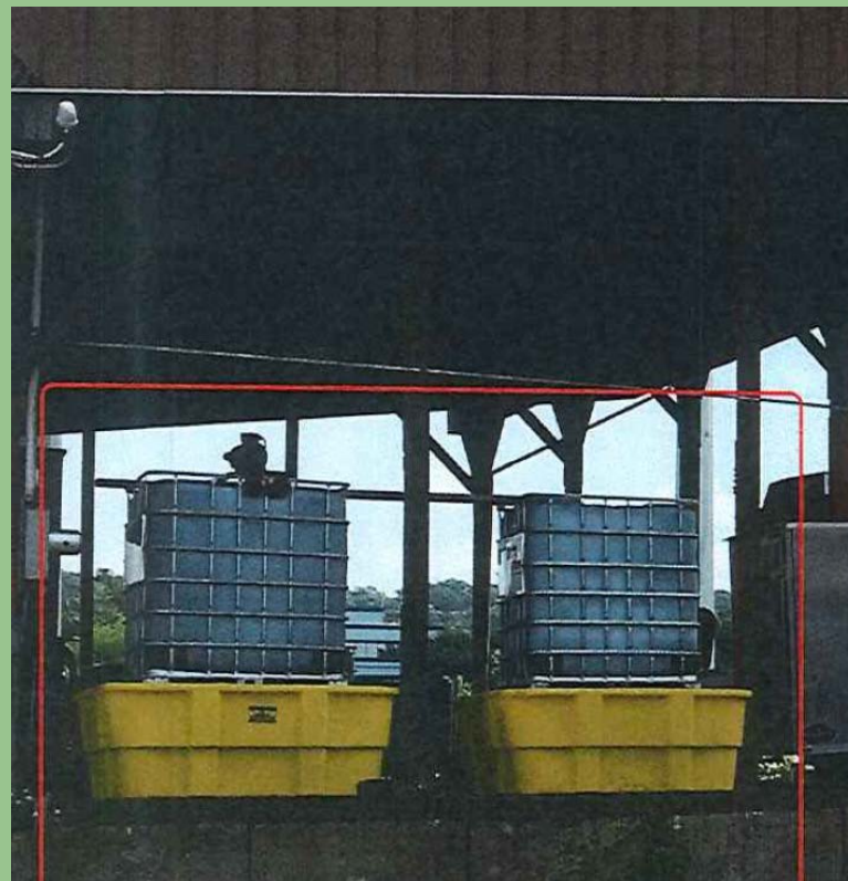
Chemical storage with secondary containment and cover
